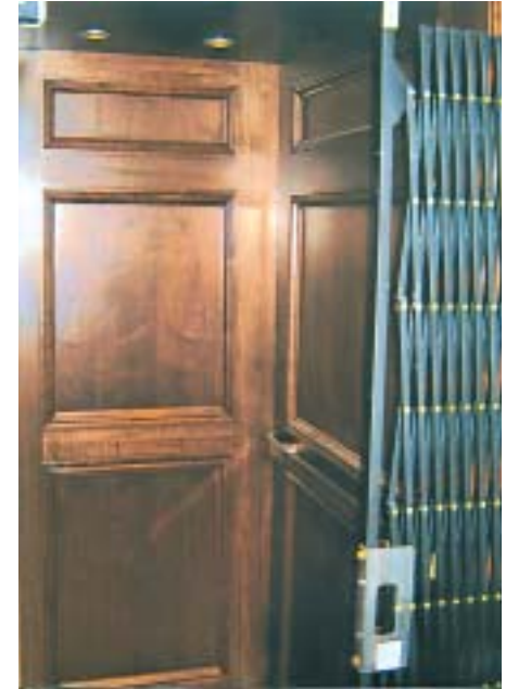
Stained Oak recessed panels with scissor gate.
